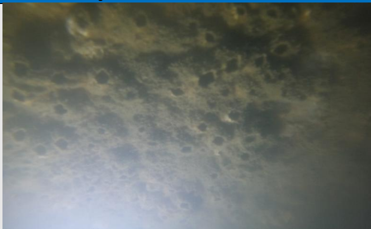
Image 2: Pile P-09 Below tide level covered largely by organisms.
