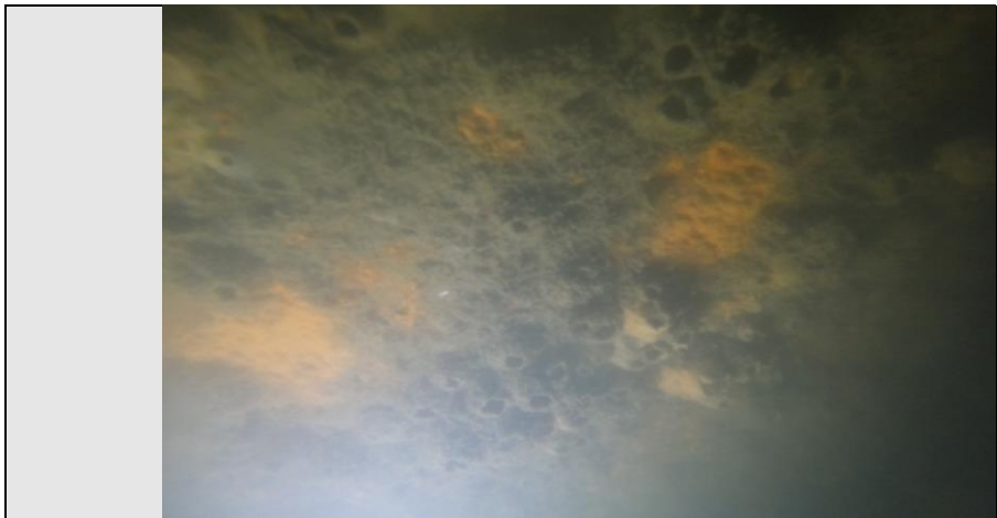
Image 3: Pile P-09 covered by marine organisms and corrosion on patches.
