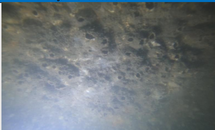
Image 2: Pile P-07 Below tide level covered largely by organisms.
