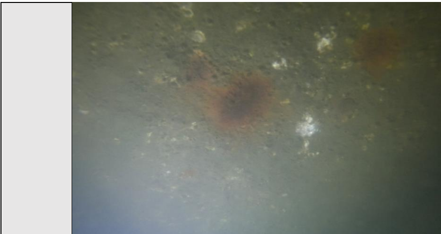
Image 3: Pile P-06 covered by marine organisms and corrosion on patches.
