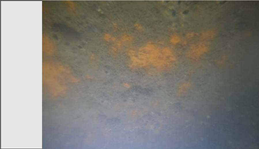
Image 4: Pile P-06 metal expose with presence of corrosion and porosity.
