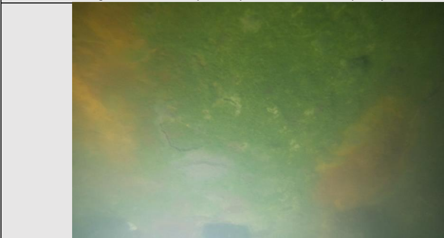
Image 5: Pile P-06 metal expose with presence of corrosion and porosity.
