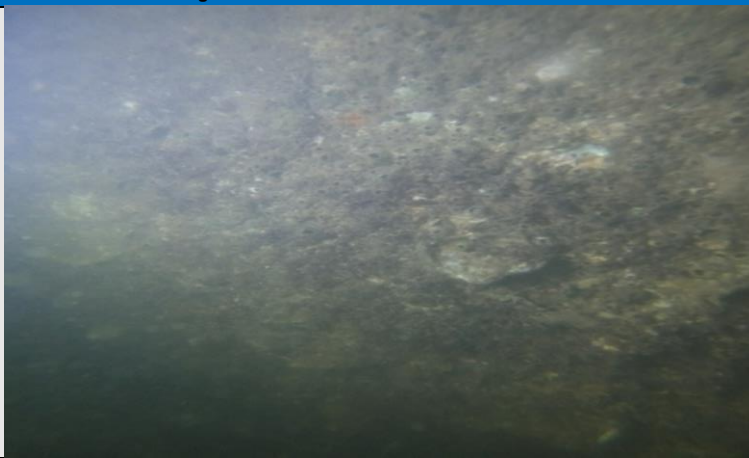
Image 2: Pile P-04 Below tide level covered largely by organisms.
