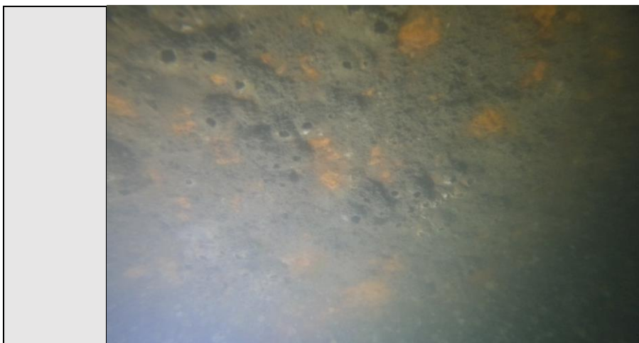
Image 3: Pile P-04 covered by marine organisms and corrosion on patches.
