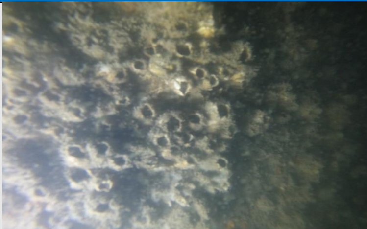
Image 2: Pile P-03 Below tide level covered largely by organisms.
