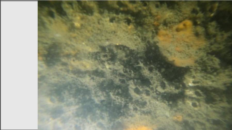
Image 4: Pile P-03 metal expose with presence of corrosion and porosity.
