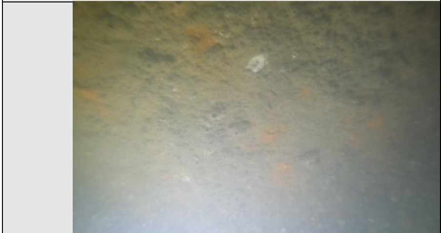
Image 4: Pile P-02 metal expose with presence of corrosion.
