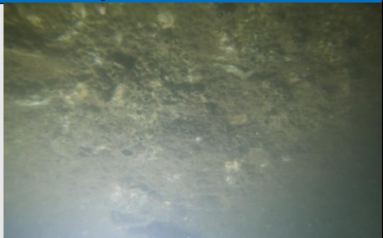
Image 2: Pile P-02 Below tide level covered largely by organisms.
