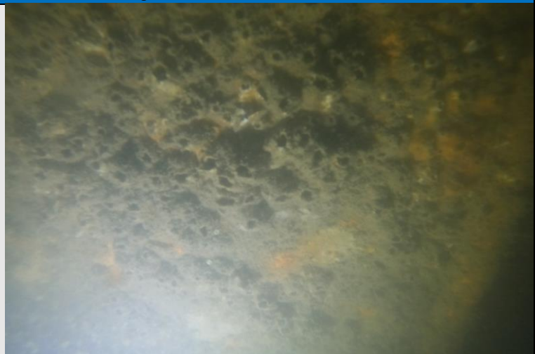
Image 2: Pile P-01 Below tide level covered largely by organisms.
